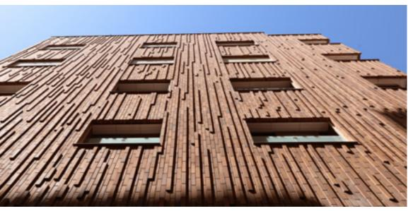
Brick veneer is a non-structural layer of brick used in construction of buildings, placed at outer layer, generally backed by an air space. The materials used in brick masonry work and that in brick veneer are same, however, they differ in the construction technique used while placing bricks. In case of brick veneer, inner layer may be that of wood, metal or concrete. Before we move into the topic, it is necessary to understand the fine difference between Brick veneer and brick masonry work.
