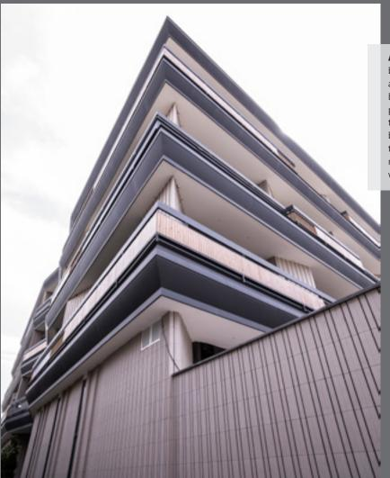
**Azarakhsh** brick facade gives beauty and delight to the appearance and ultimately is a suitable view for our building. **Azarakhsh** facade firebrick plays the role of heat and cold resistance that prevents waste of energy produced by heat and cold systems. Depending on the material color, and exposure surface it reflex the sun heat on summers and vice versa in winter.
